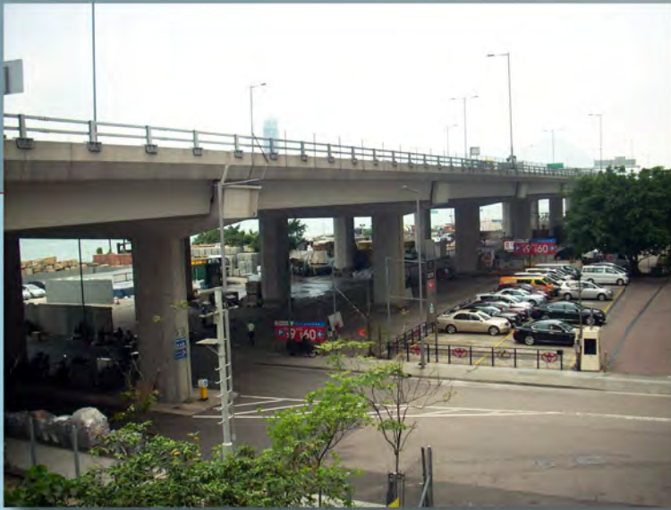
Existing Condition Under the IEC Bridges
